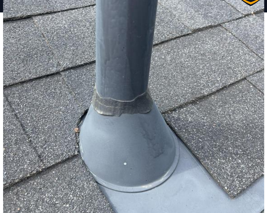
Properly sealed and installed vents
