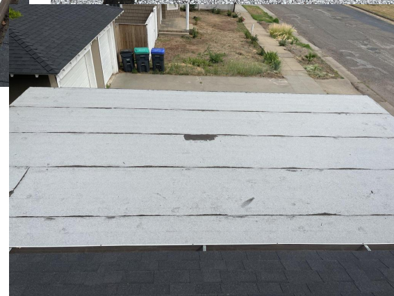
Missing granules. Previous repairs visible.
