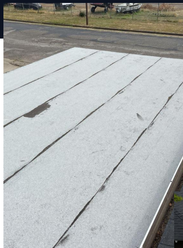
Missing granules. Previous repairs visible.
