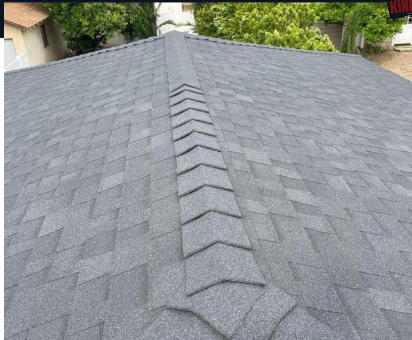
10 Inch Bull Nose Ridge Cap - No Ridge Vent
